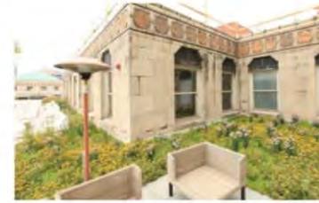
GREEN ROOF OUTDOOR RESIDENTIAL TERRACE
