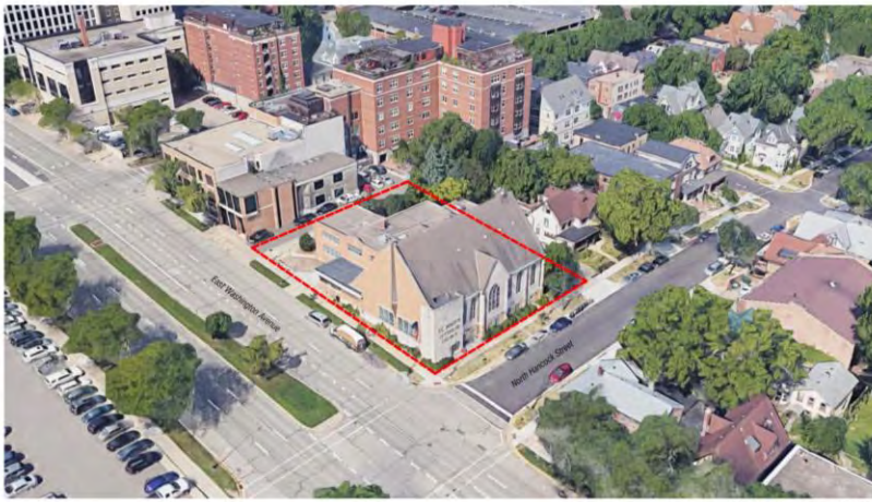
332 East Washington Avenue - Existing Site
