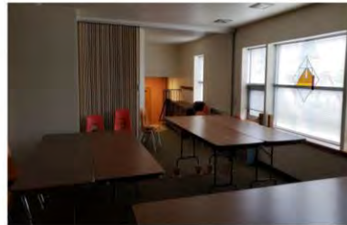
Existing Interior Image
